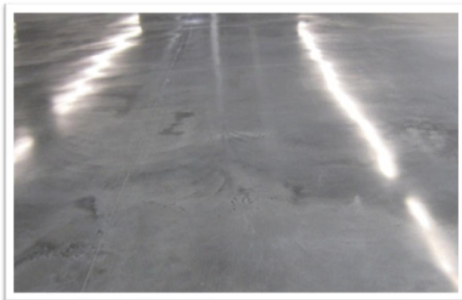
This type of floor has lower resistance to abrasion and a relatively shorter lifetime. It can be used for areas with light foot traffic, requires repeated application of impregnating sealer after a certain period of time.
